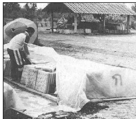
An easy-access curing chamber can be stepped into.
