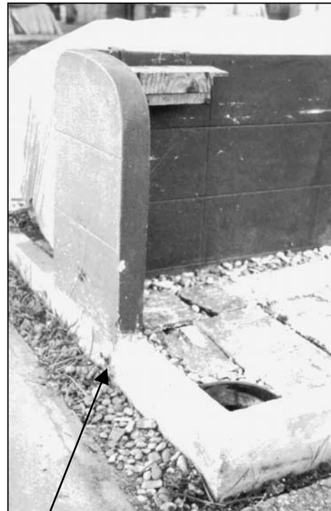
An overflow pipe helps prevent liquid water from touching the concrete products and causing efflorescence.
